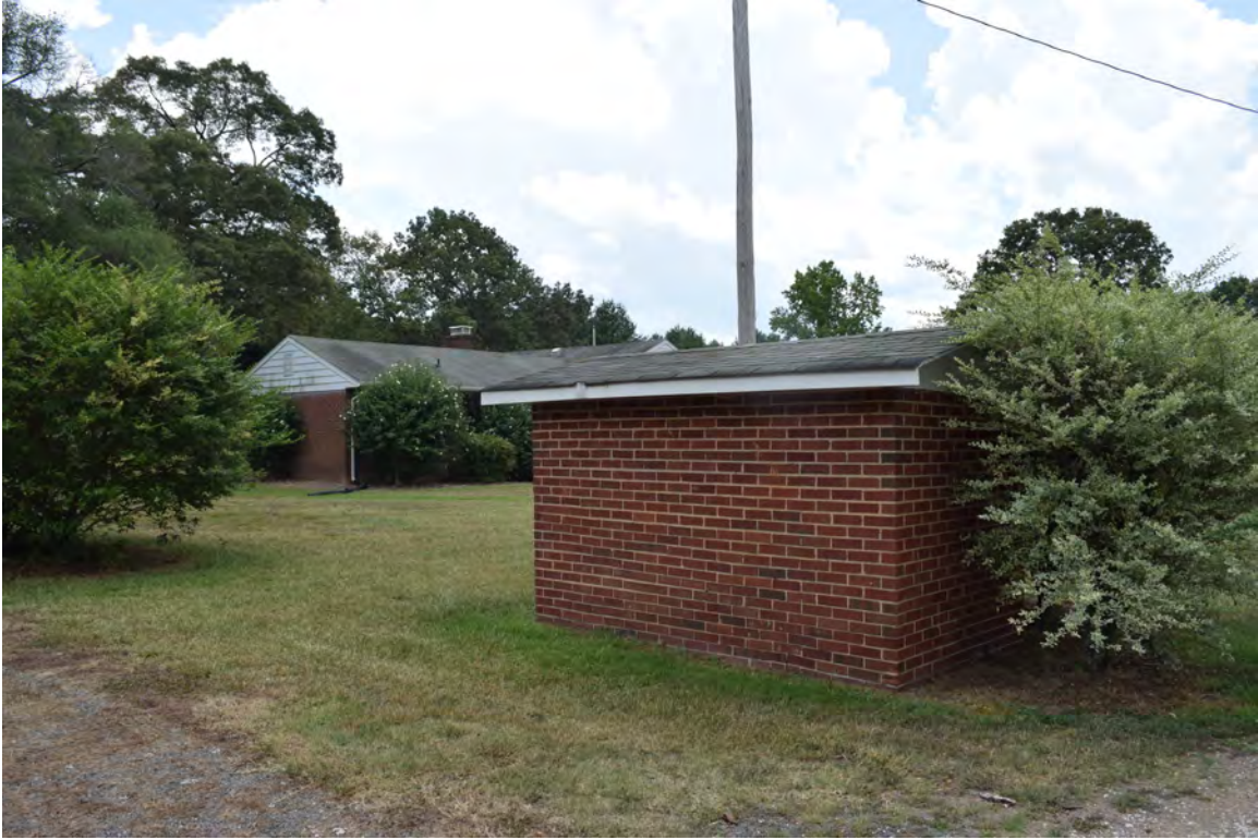
Figure 12: Brick pump house northwest of the manse, view to the southeast
