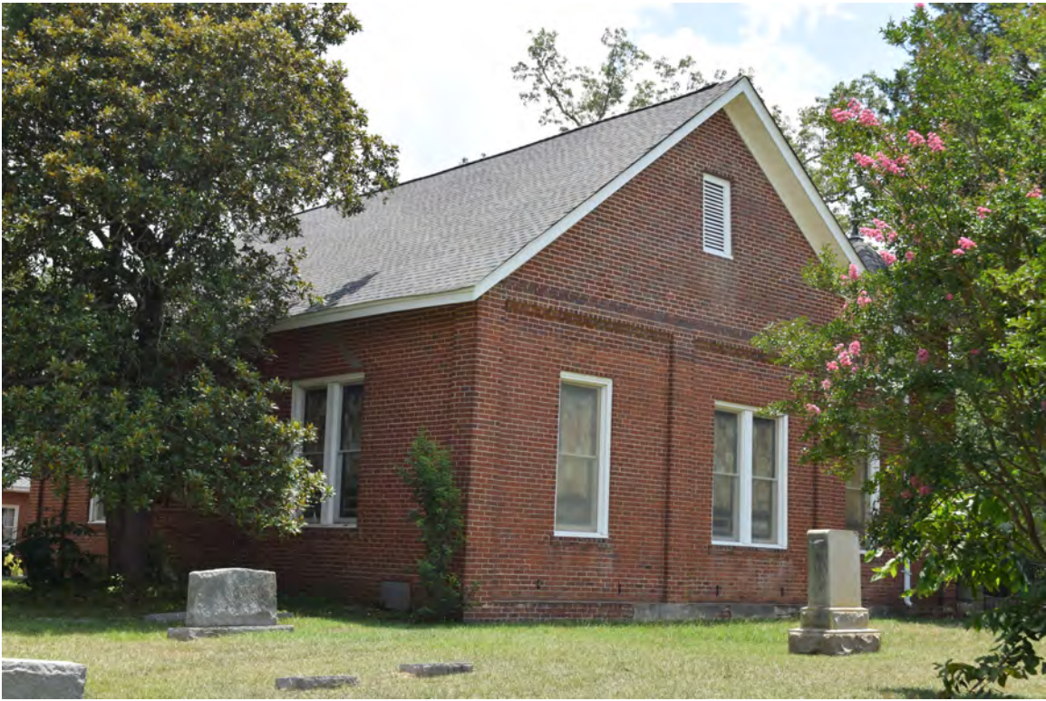
Figure 35: Northwest corner of church, view to the southeast
