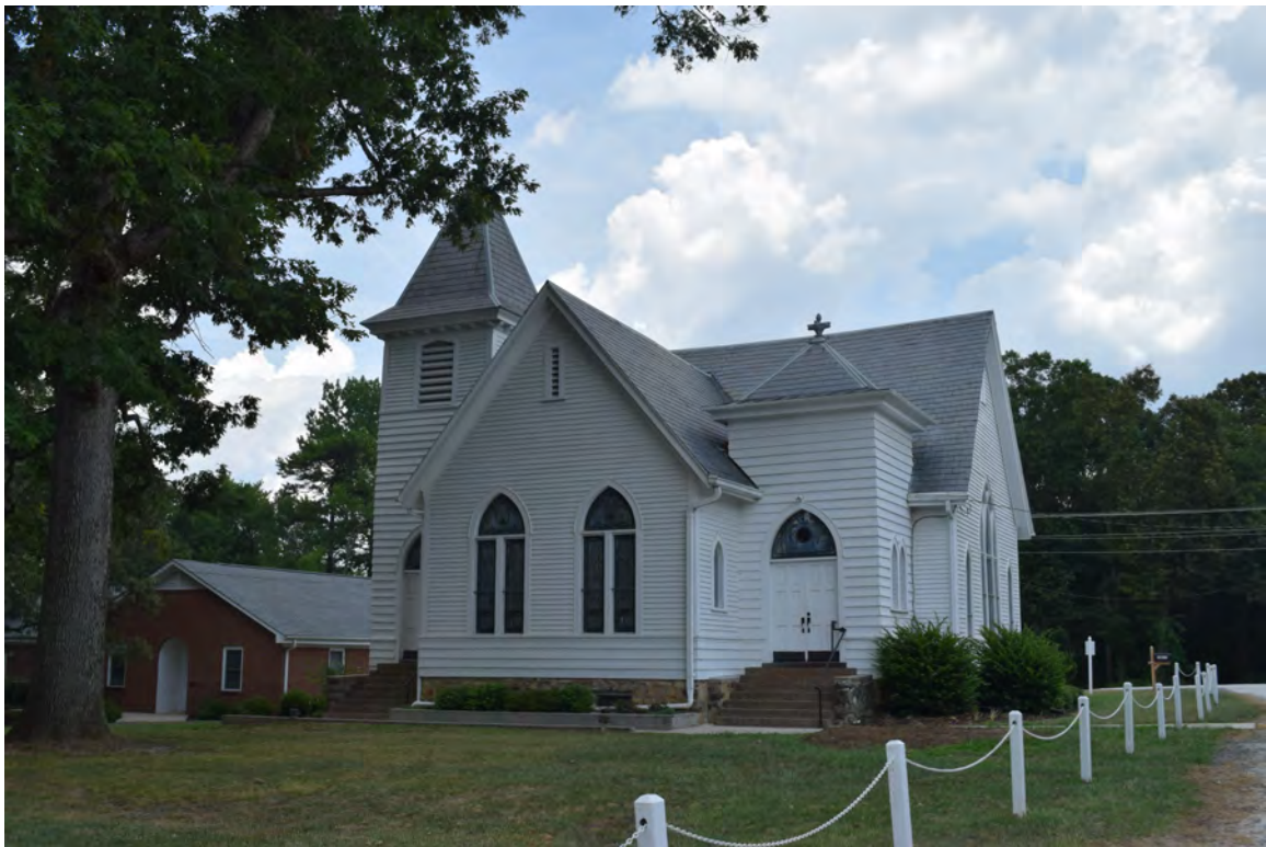
Figure 7: Southeast corner of Banks Presbyterian Church, view to the north-northwest
