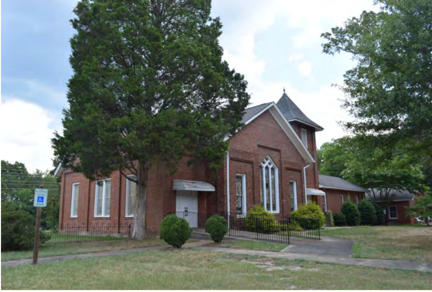
Figure 49: Marvin United Methodist Church, view to the northeast
