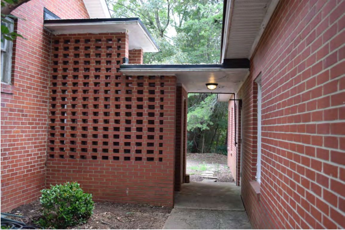
Figure 38: Space between Sunday school wing (left) and fellowship hall, view to the north
