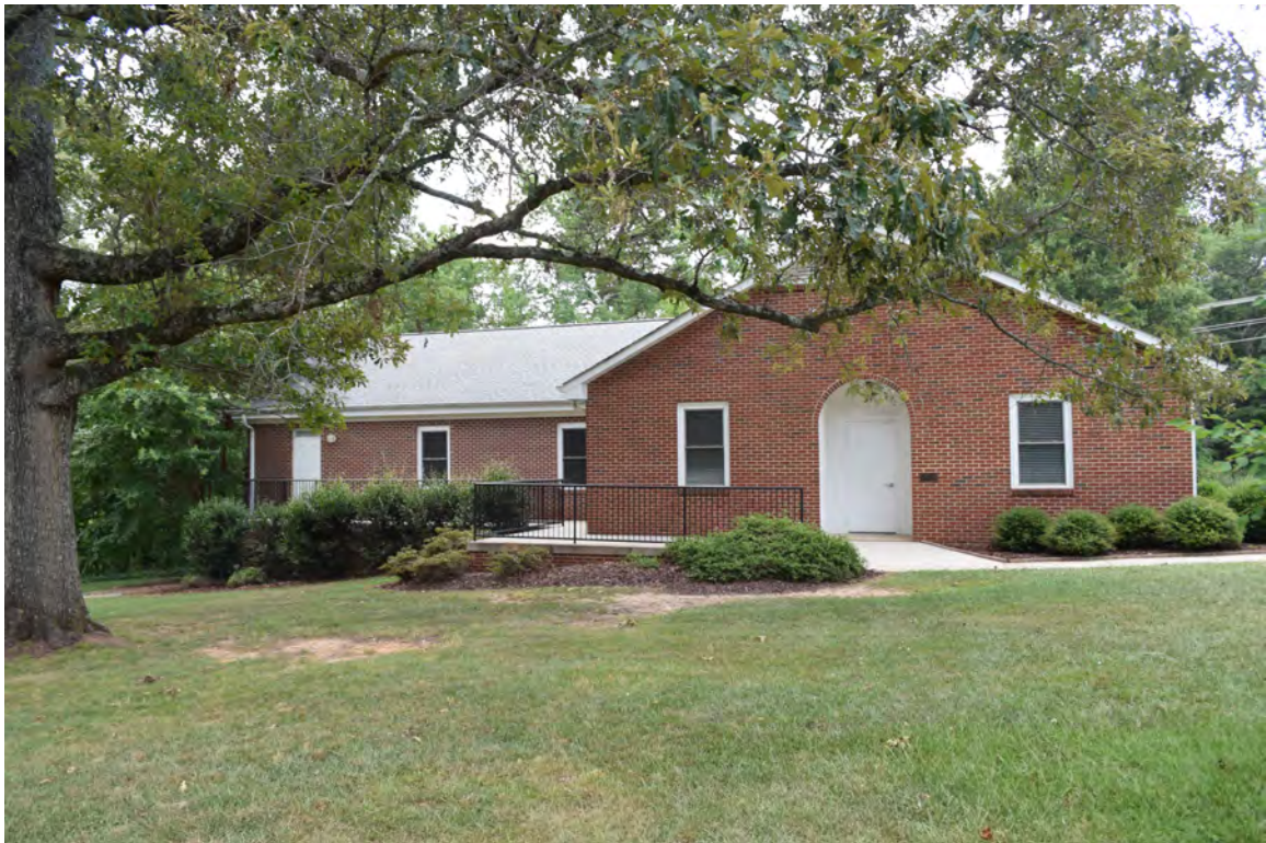
Figure 8: 1961/2004 fellowship hall, south elevation, view to the north
