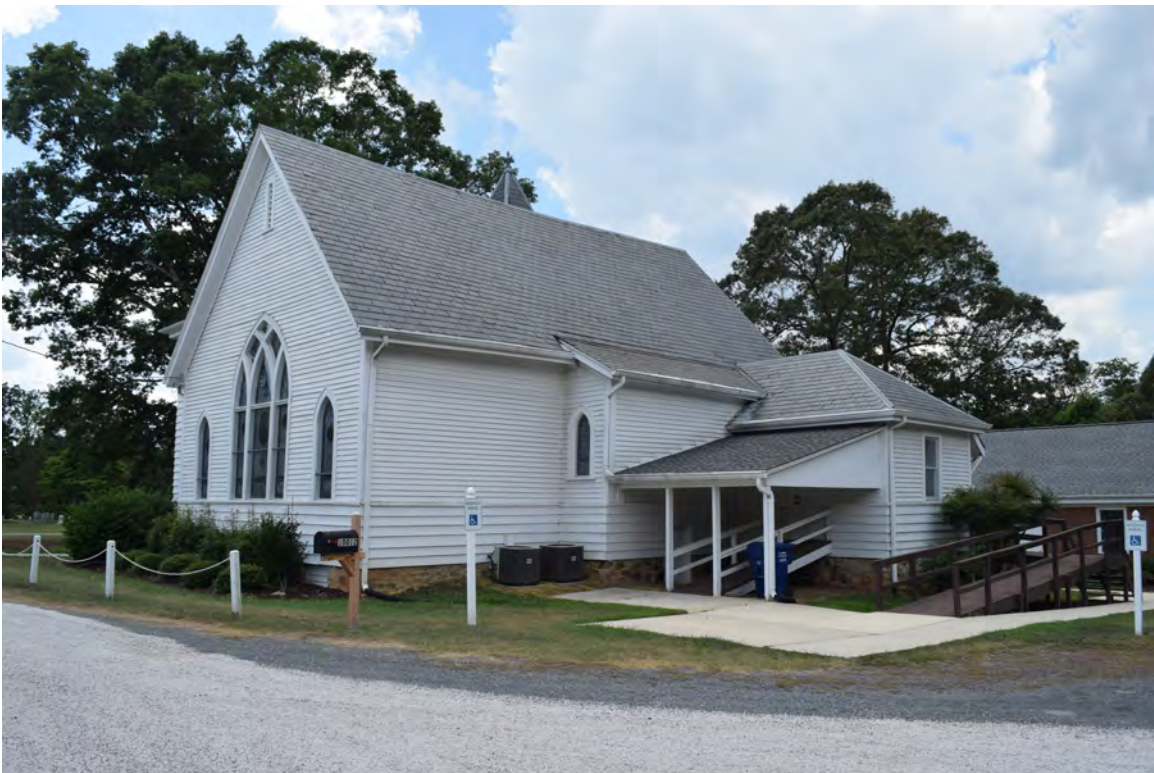
Figure 11: Northeast corner, view to the southwest
