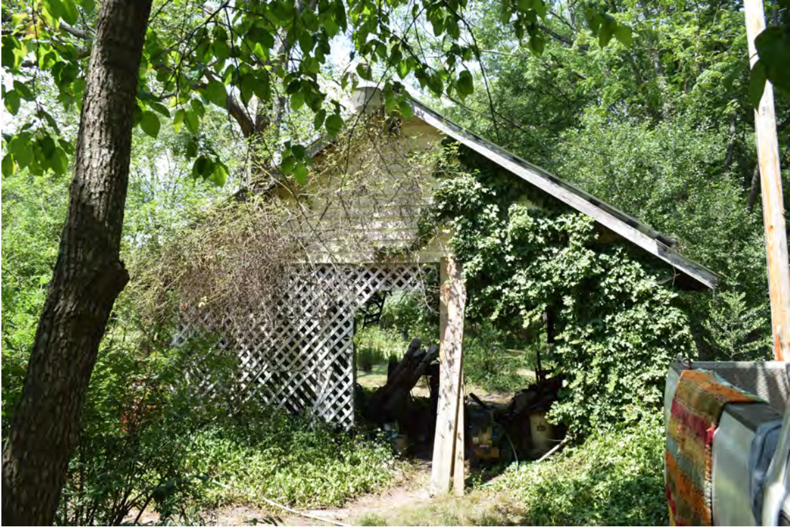
Figure 26: Garage, view to the north
