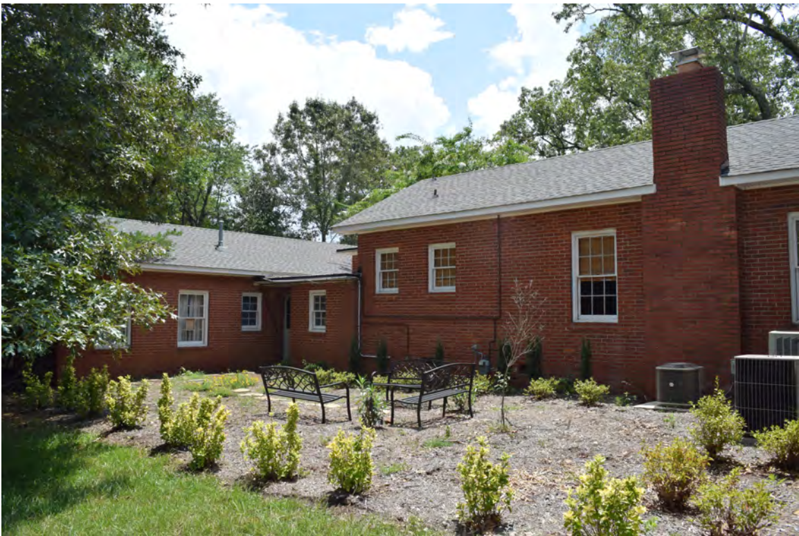
Figure 37: Rear of Sunday school wing and west elevation of fellowship hall
