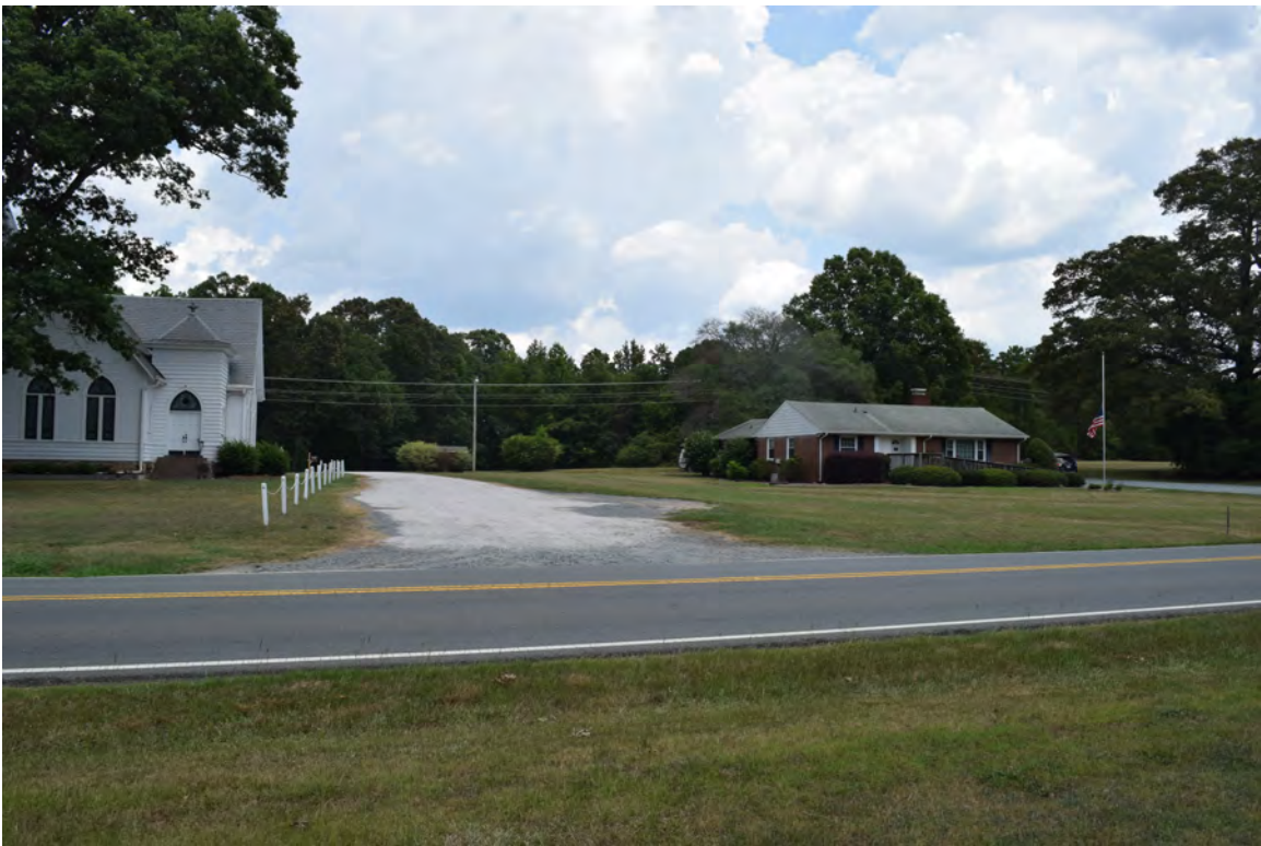
Figure 13: Manse with church to the west, view to the north-northeast
