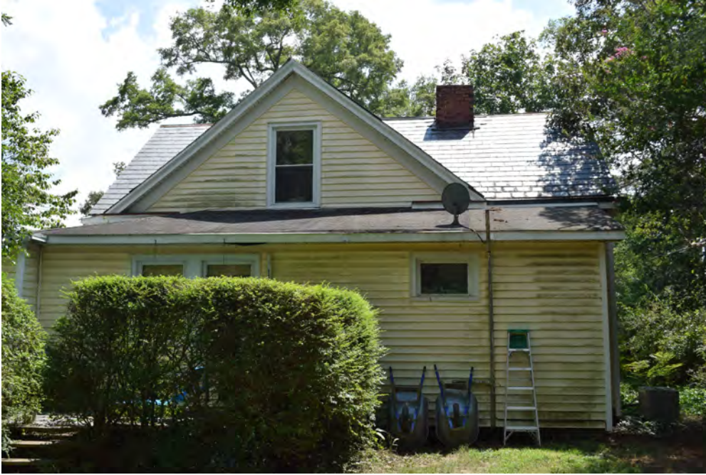
Figure 24: Frank S. Crane House rear elevation, view to the south
