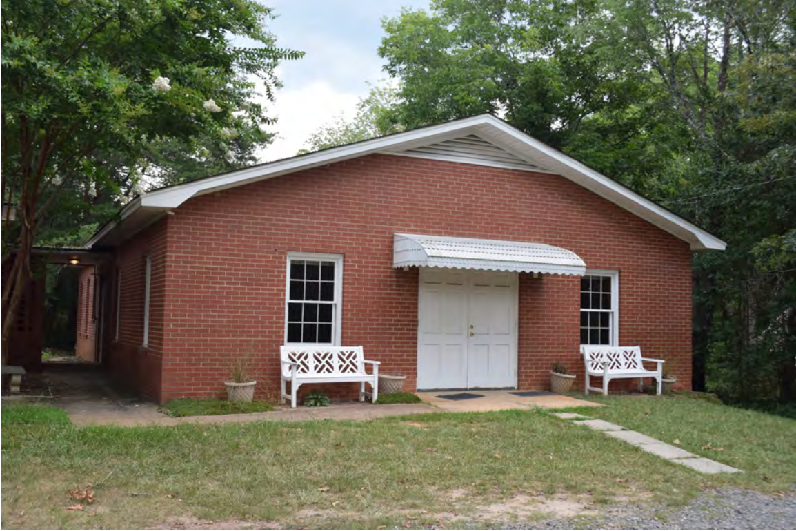
Figure 36: 1967 Fellowship hall, facade, view to the northeast
