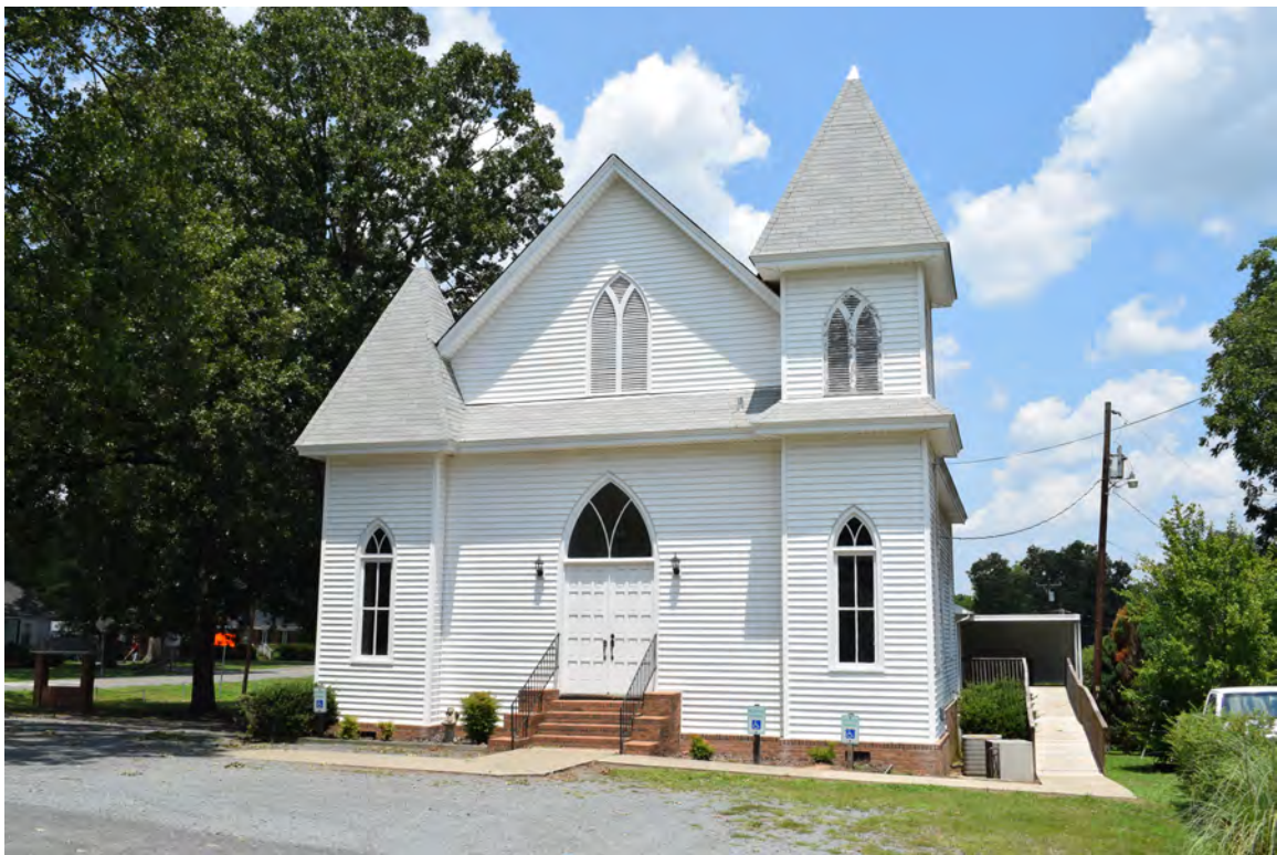
Figure 19: Unionville Methodist Church (UN0404)
