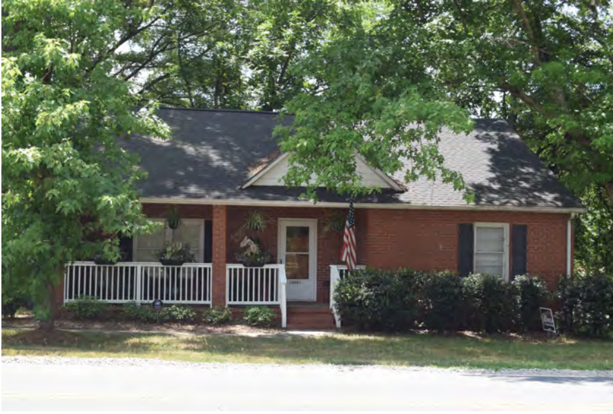
Figure 48: William and Willa Crane House, view to the south
